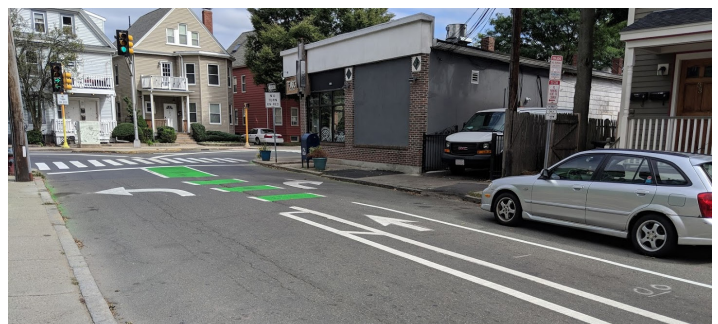
Northbound buffered bike lane on Cutter Ave.
