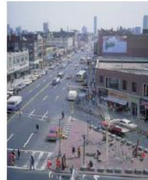
Before improvements were made, Massachusetts Avenue had the character of a highway. Pedestrian crossings were very hazardous and there were no provisions for bicyclists.
