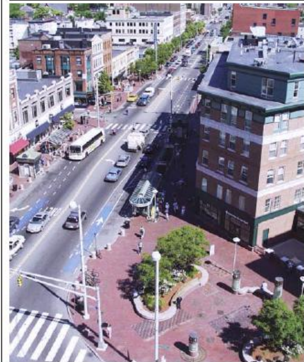
The improved public realm in Central Square, with Carl Baron Plaza in the foreground. Sidewalks were widened and pedestrian crossings were clearly delineated. Bicycle lanes were provided.
